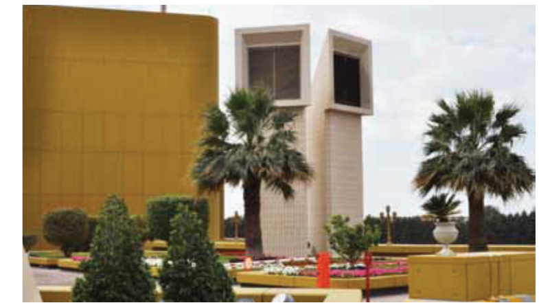
Inaccessible infrastructure opening
