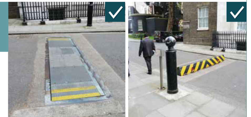
Effective adaptable measures to control access of vehicles (Downing Street, London, UK)
