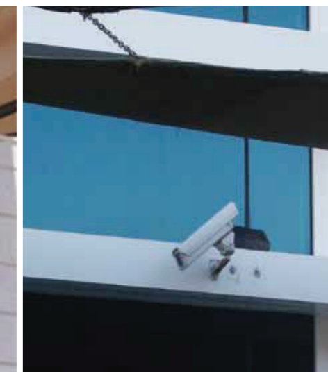
At these buildings in Abu Dhabi, CCTV cameras have been installed below shading canopies
