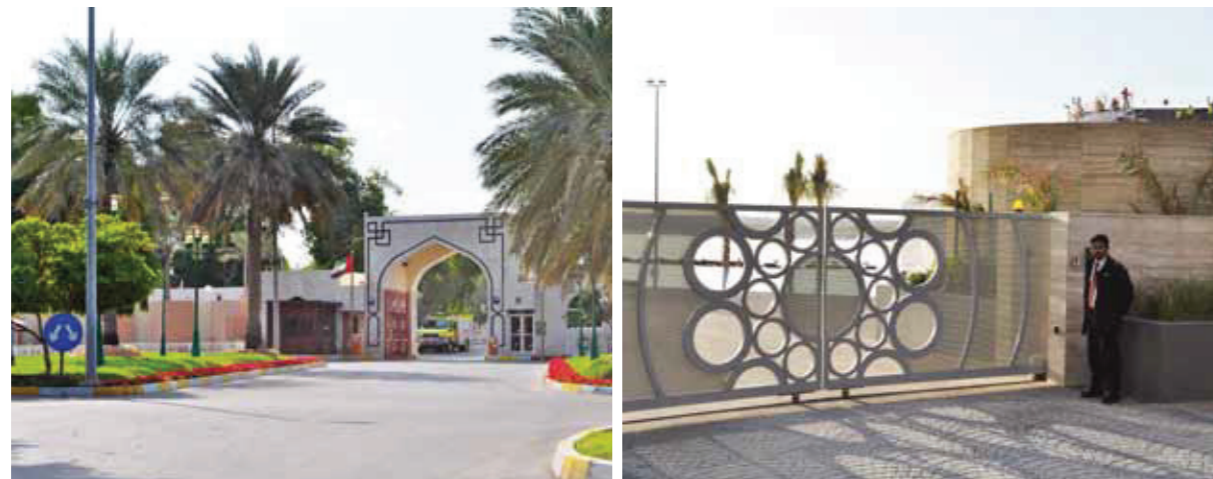
Typical vehicle access control points at existing developments in Abu Dhabi
