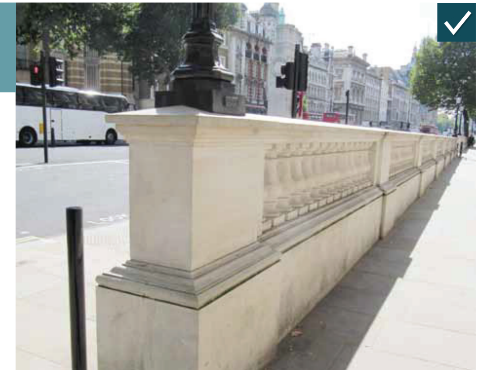
This ornate wall has been specifically designed to provide hostile vehicle mitigation and to match the context of the surrounding environment (London, UK)
