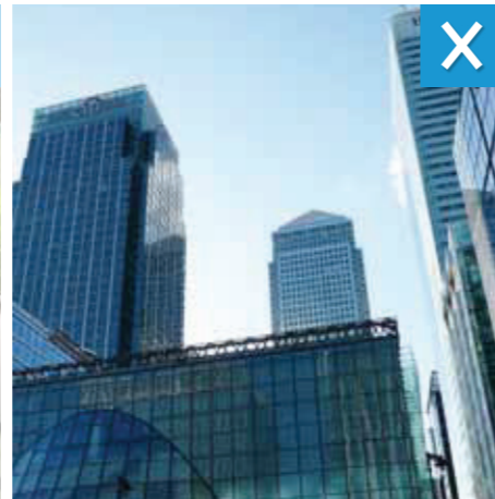
The designers choice of glazing could result in secondary fragmentation risk in a crowded place
