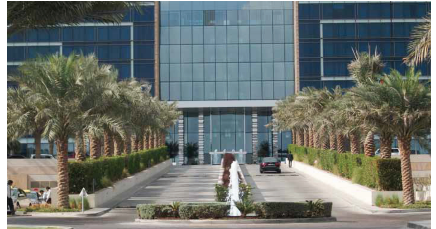
This existing building is set-back from the street. It would be relatively simple to introduce stand-off if deemed necessary
